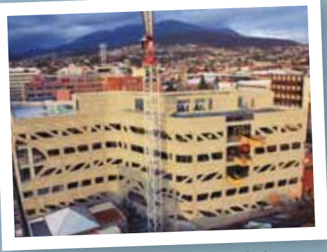
Progress shot of the new UTAS Medical Sciences building, Hobart (March 2009).
