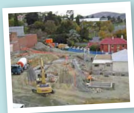
Laying a solid foundation
