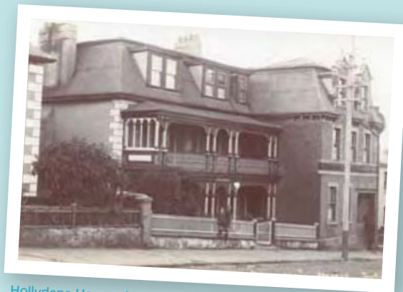
Hollydene House shortly after the 1909 additions had been completed
